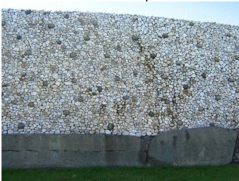
The masonry of the stone layers is very intricate. The quartz stones are an outside finishing layer, in
