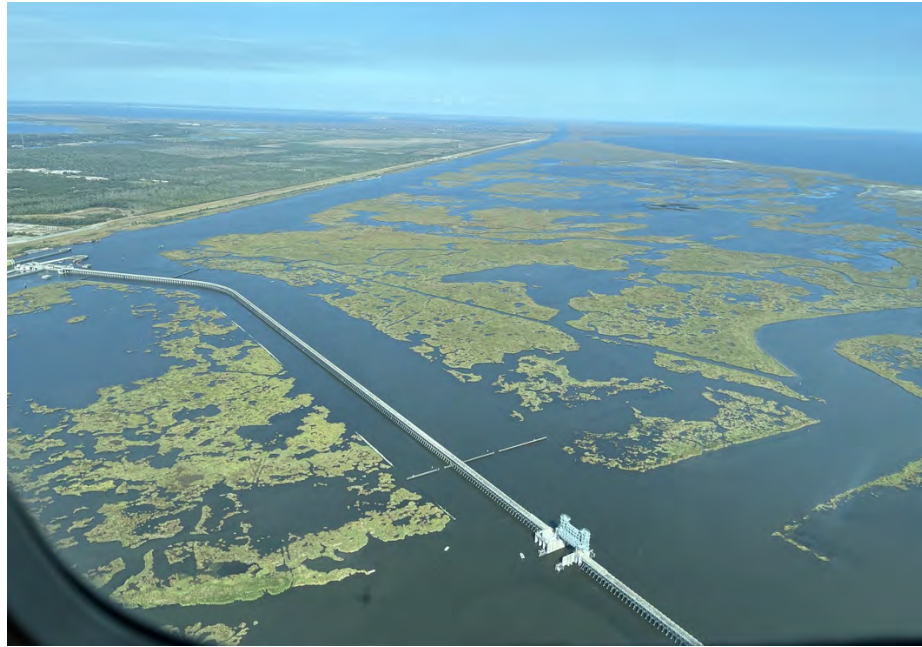
1.8-mile Lake Borgne Surge Barrier with Bayou Bienvenue Vertical Liftgate. Gate on far left is Gulf Intracoastal Waterway Barge Gate. View from author's Mississippi Delta sea plane flight. Photo by author.
