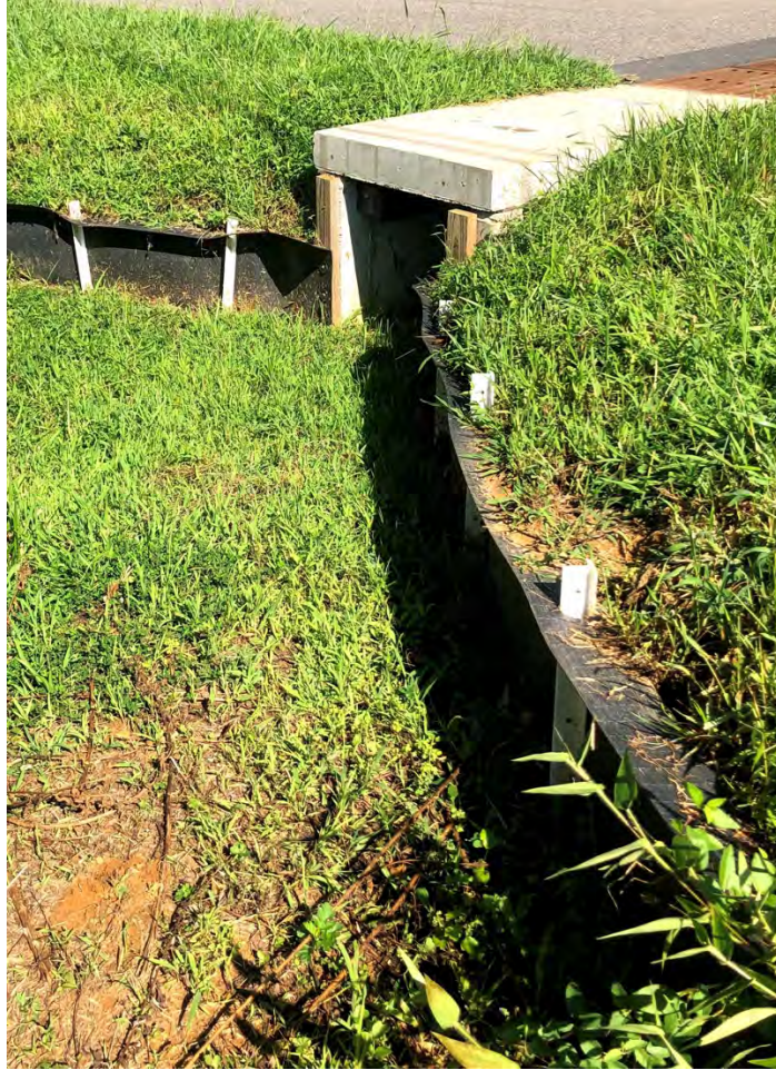
Entrance for a turtle passage system beneath a roadway. Photo: NJ Division of Fish and Wildlife.
