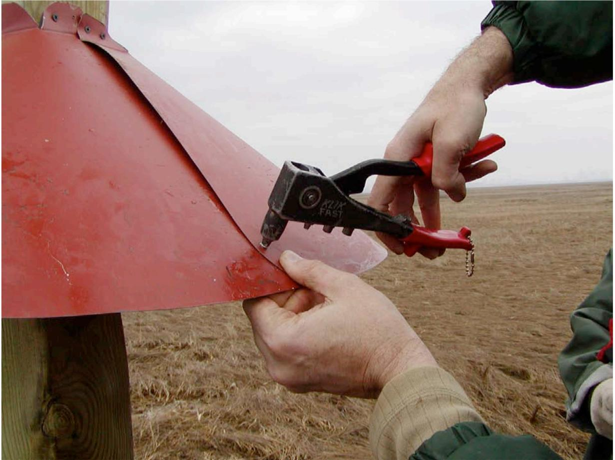
**Inserting pop rivets in holes**
