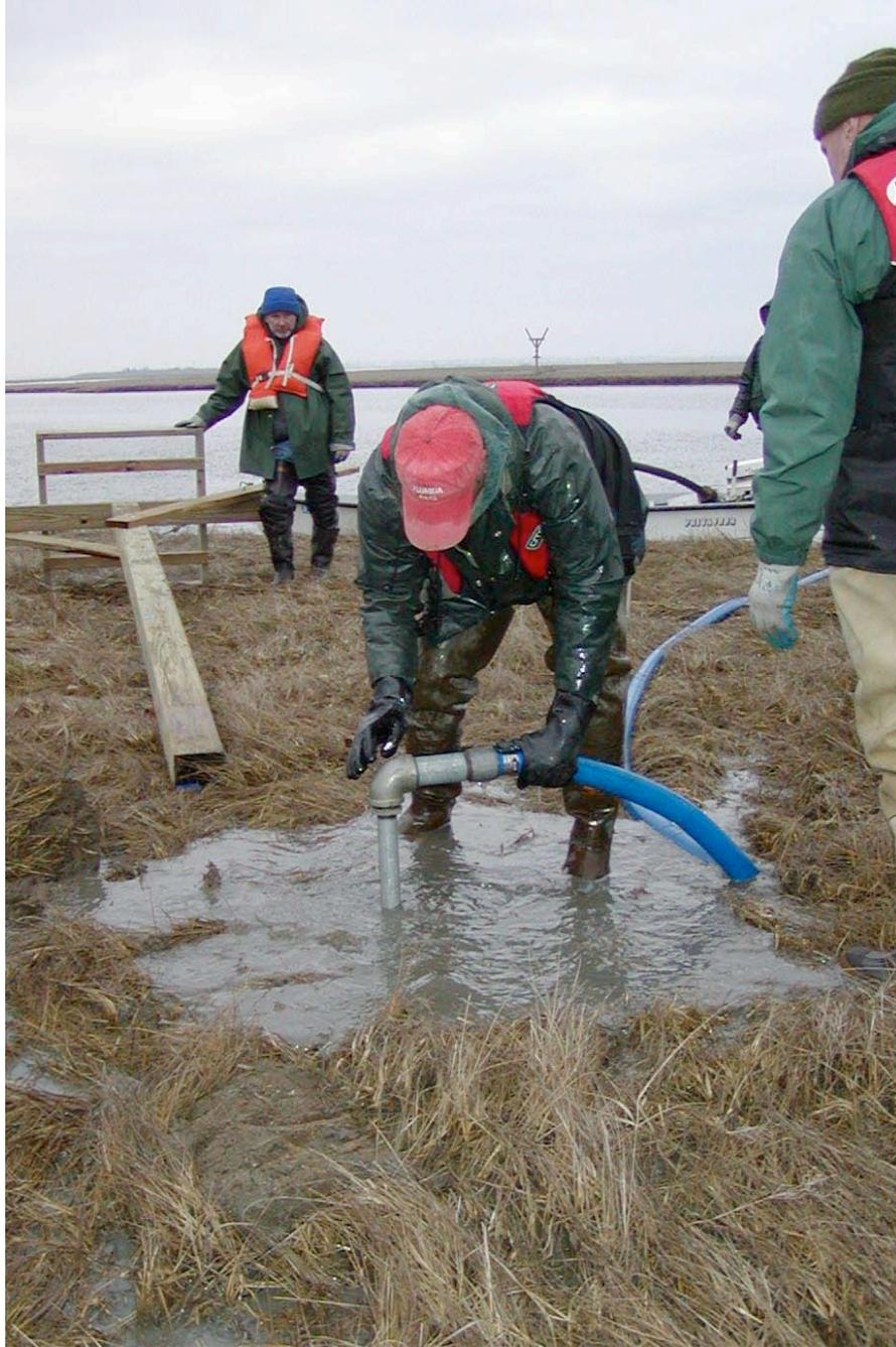
When the hole has reached about 5-6 feet deep, we allow the water to run until it seems as though the hole is the proper circumference to take the pole. The individual who is handling the pipe will wiggle it around to get a sense of this.
