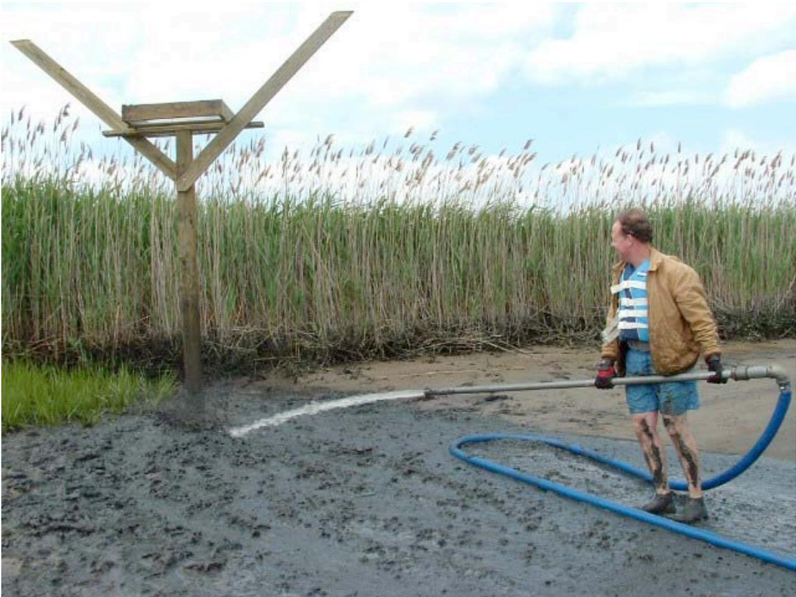
If the pole is too loose once it is in place, it may help to backwash the nest from a bit of a distance, as in the above photograph. Often we tamp the dirt in around the pole with our feet, but this approach can seriously twist an ankle and should be done only by a person with proper boots and good physical abilities.
