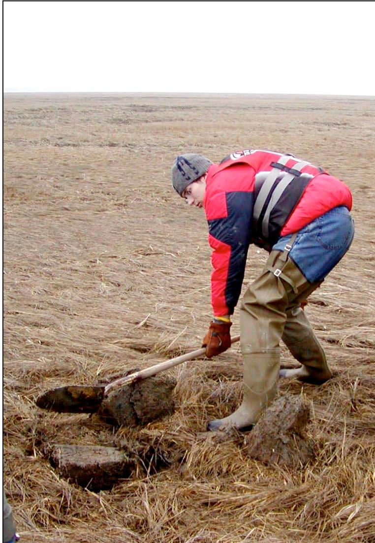
Once we have arrived at the erection site, we break the surface of the marsh with a shovel if there is a thick mat of vegetation that needs to be removed in order to jet a hole in with water. On the Maurice River, we normally have a sandy or muddy surface and this step is not normally necessary. But where you have cord grass/ *Spartina alterniflora* or *patens* you will want a shovel as part of your arsenal.
