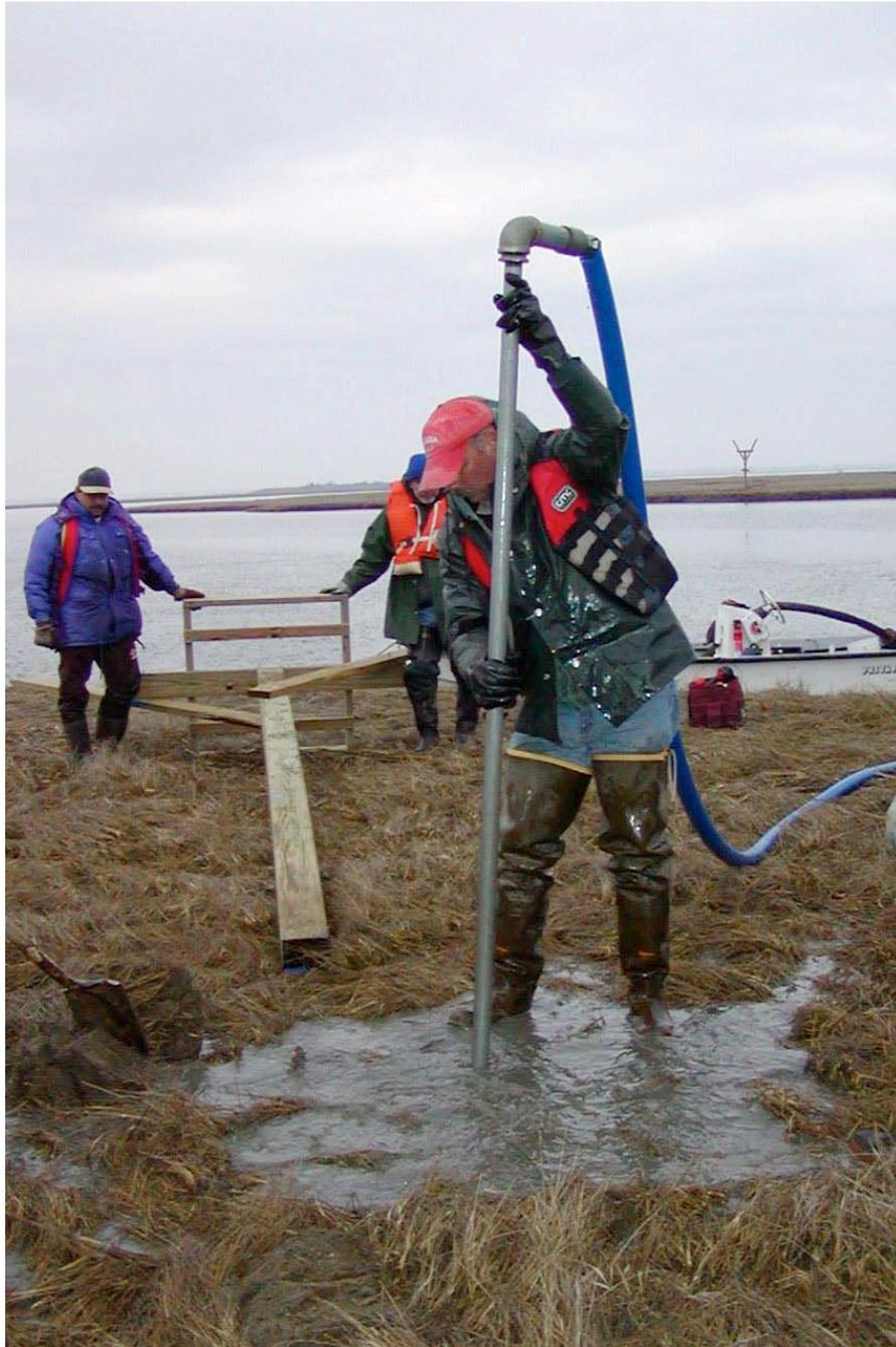
Allow the pipe to wash in a hole large enough to accommodate the 6-inch square pole. We prefer this to using a post-hole digger. If you hit a hard object, it may be preferable to move a few feet away. But it is wise not to allow this hole to be in the path of those erecting in a different hole. Marsh plains in our area are already ankle twisters due to rough terrain and muskrat tunnels.
